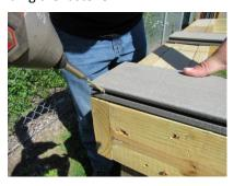
When using fasteners, always be sure to leave a 3/4" gap between the fastener and the end of the Plank.
