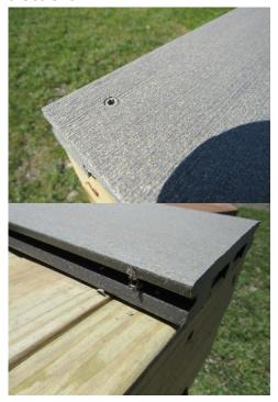
3. Install subsequent planks while being sure to maintain a 3/16" gap between planks and other obstructions such as posts and walls.
