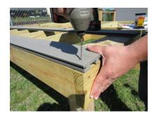
b. #7, #8 or #9 x 1-5/8" stainless steel or coated "trim head" screws can be driven at a 50-60 degree angle thereby hiding the fastener.
