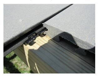
3. Leave a 3/16" gap at the butt joint to allow for expansion and contractions of the planks.
