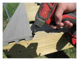
c. Angle the next plank as shown below and apply pressure to slide the plank into place.
