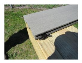
Secure a clip into each joist with the provided screws. The screw should be driven through the guide hole at a 45 degree angle.
